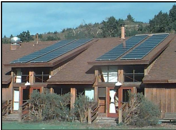
Solar PV systems at NPS lodging (Photo courtesy of Steve Butterworth)
